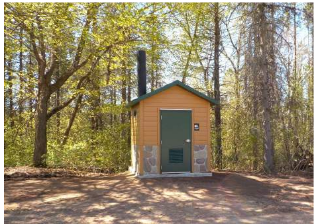
New handicapped accessible restroom
