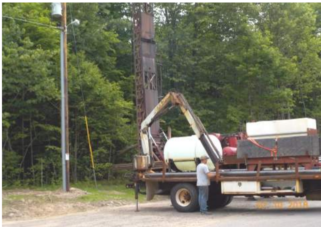
Drilling new well
